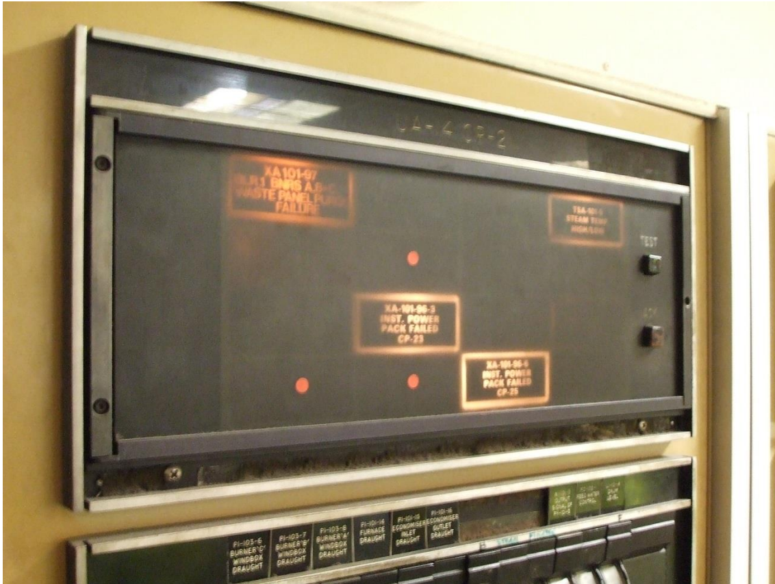
Old alarm system
